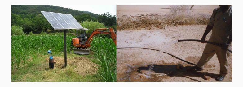
SOLARWATER is a submersible continuous current pump – low power and high performance pump that may be fed with 24V and 48V, with current absorption of 1A and 6A adapted to the pumping heads of (10 to 175 meters).
